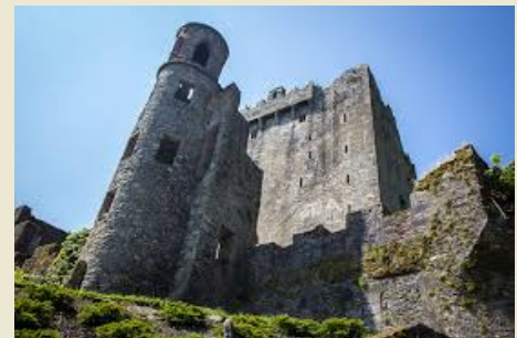
Blarney Castle - The original stone fortification, built around 1210, was destroyed in 1446, but rebuilt by Cormac Laidir MacCarthy
